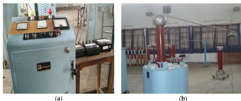
Figure 1. Experimental setup. (a) Control panel; (b) Transformer connection.
