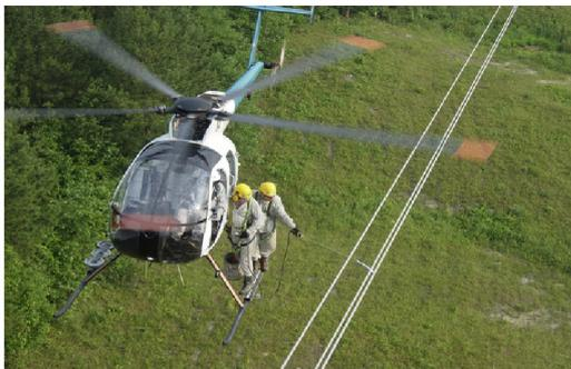
Figure 1.1: Power Line Inspection using Helicopter *Image credit:* [37]
