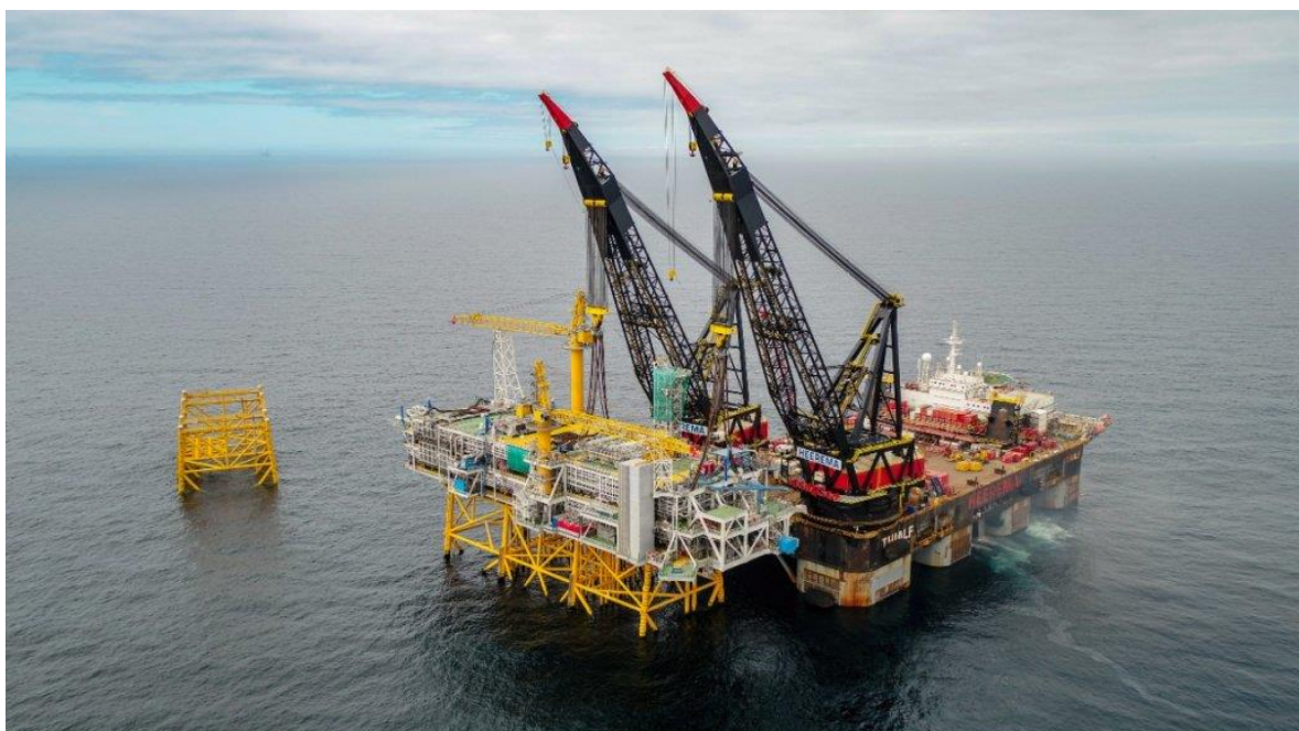
Figure 3-3 Offshore hook-up and completion: The last module of the Johan Sverdrup riser platform lifted into place April 2018 by the heavy-lift vessel "Thialf". (Equinor, 2018) .
